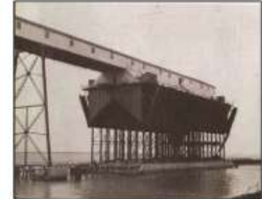
Quarry mining and shipping at Rockport began in 1914 and continued until the location was closed in 1948. Very little remains of the many buildings from the operation. A few pieces of steel beams remain. At left is a picture of the pier dock; ca. 1940.
